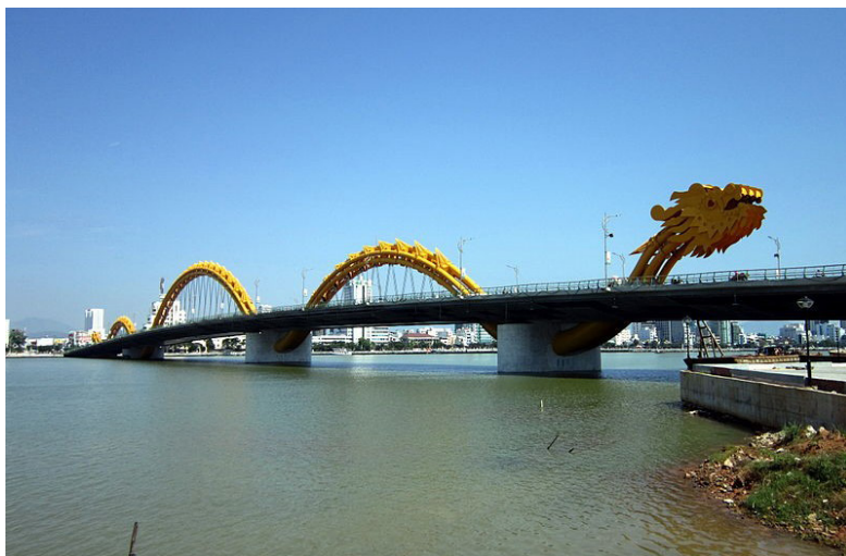
The Dragon Bridge in Vietnam uses arches that look like a dragon. Credit: Bùi Thụy Đào Nguyên/Wikimedia Commons.
